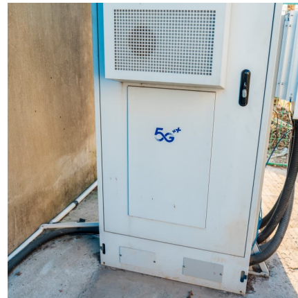
Cornerstone Electrical Supply , Vega Baja
