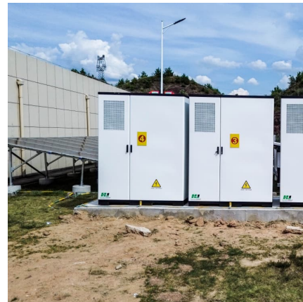
Energy storage cabinet hoisting scheme picture
