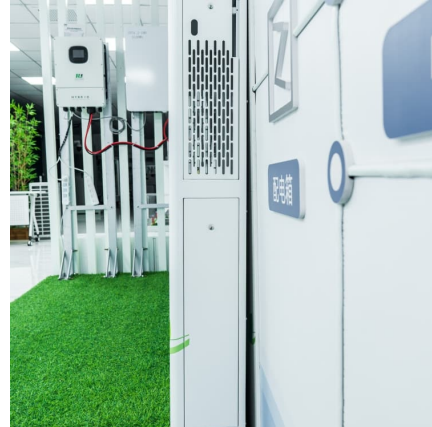
1st gravity energy storage plant , Enel Green Power
