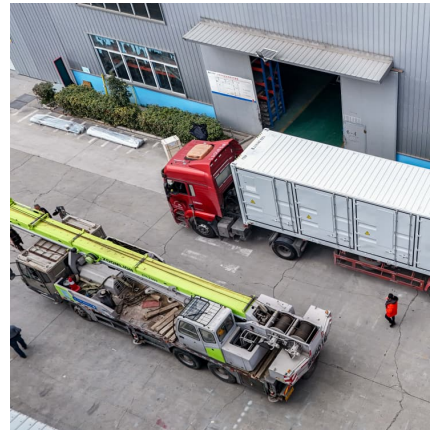
Maputo power storage vehicle source manufacturer
