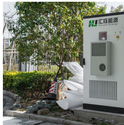
Energy Storage Cost and Performance Database
