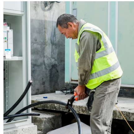
Cost Analysis: Setting Up a Lithium Ion Battery ...
