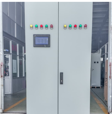
Residential Battery Storage , Electricity , 2021 , ATB
